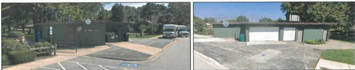
Street View - 125 East Richmond Street - Existing Maintenance Building (source: Google)
