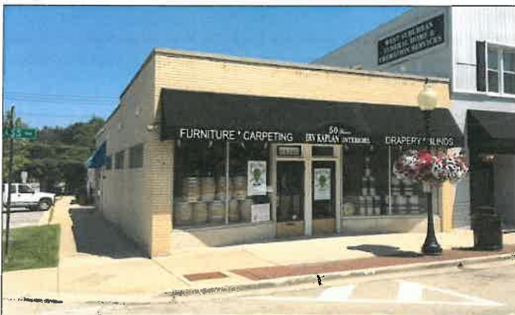
Street view - 41 North Cass Avenue
