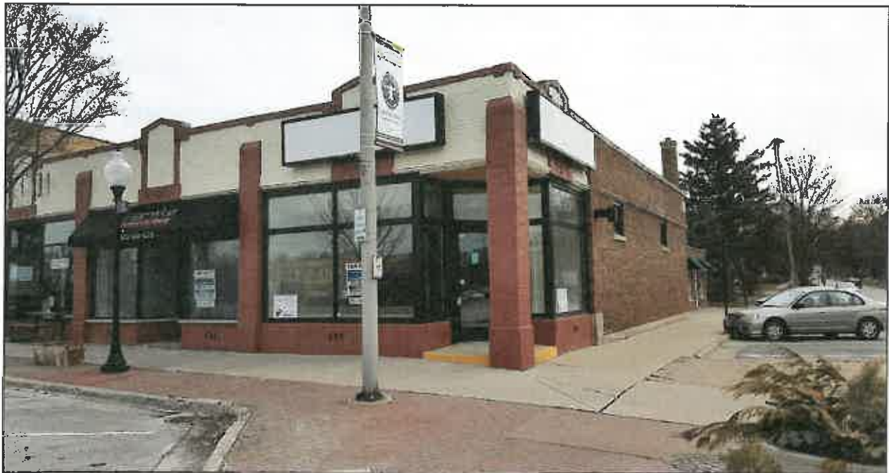
23 West Quincy Street - Storefront
