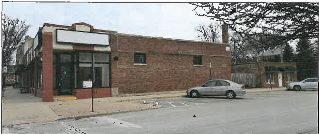
23 West Quincy Street - Adjacent parking along South Lincoln Street
